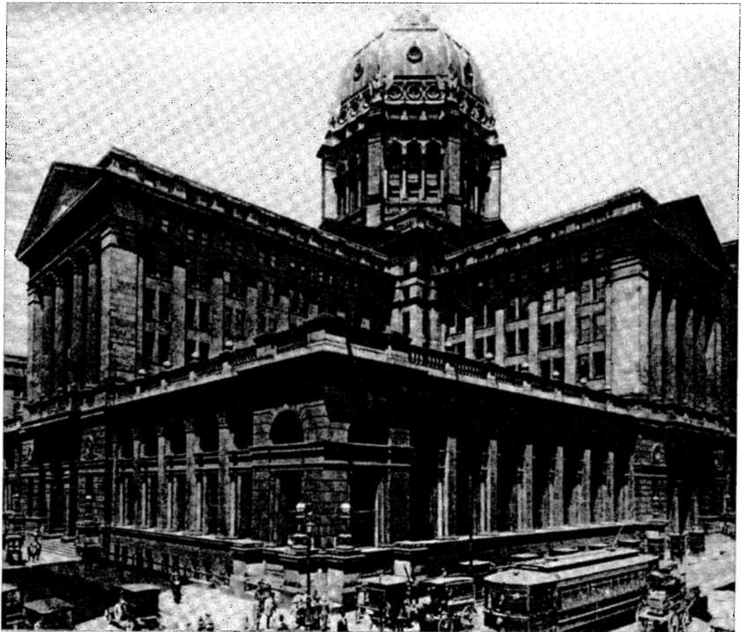
With its dramatic 300-foot high dome, the Federal Building, which Cobb designed in 1895 (completed in 1905), was one of the most cherished buildings in Chicago. It was demolished in 1965 for the current Federal Center.
